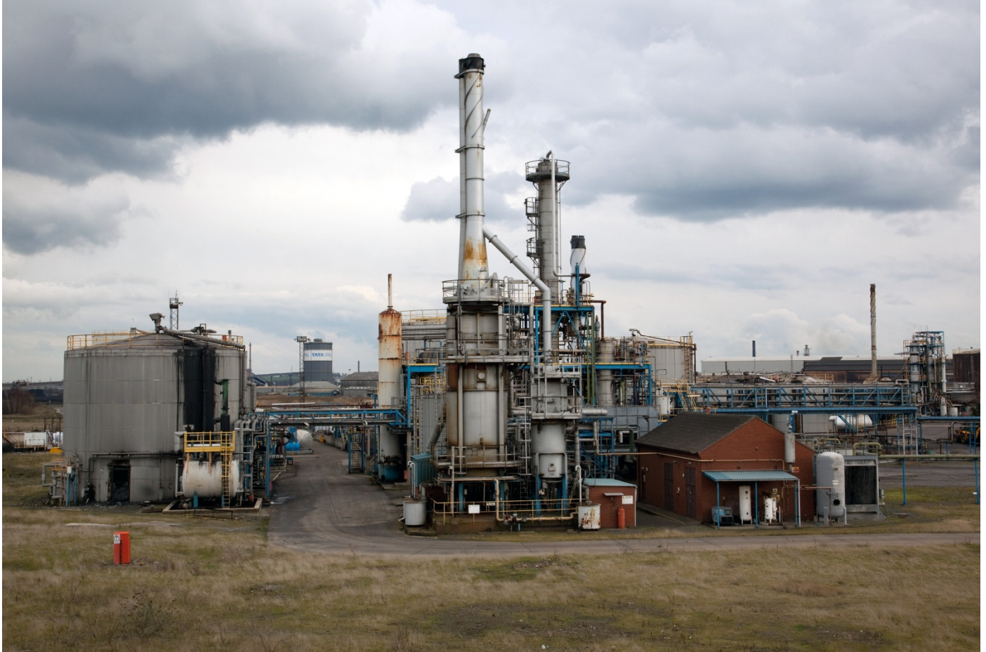
Tata Steel, Scunthorpe
